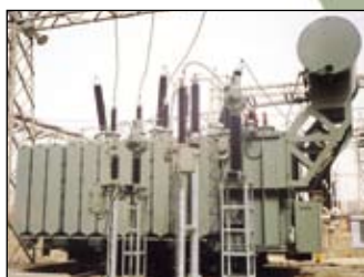
220kV 125MVA Transformer Egyptian Electricity Transmission Company in Egypt
