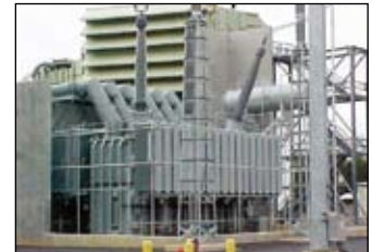
500kV 390MVA Generator Step-up Transformer Tenaska Georgia Power Plant in U.S.A.
